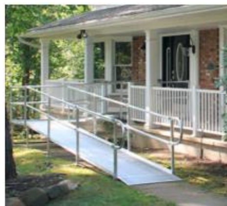
Outdoor ramp, Source: National Ramp
